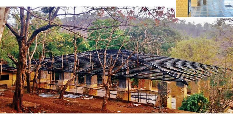
We reconstructed the new roof using steel trusses and reused the existing roof tiles. This reconstruction allowed us to slightly increase the height of the building, to remove the existing internal pillars thereby ensuring the building will better meet our needs, and will guarantee the structural integrity for many years to come.
